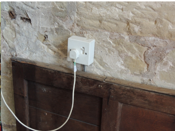
2 amp socket outlet by pulpit
