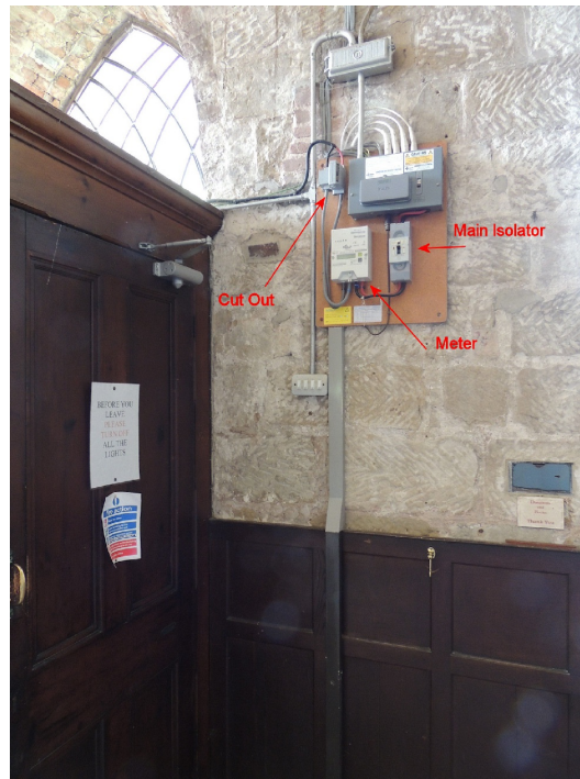
Electrical supply and fuse board
